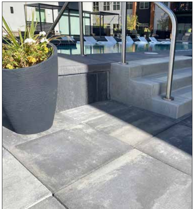
The CityStone XL paver measures 24 by 24 by 2.36 inches. The color on this project is a random blend of charcoal and slate that creates a cool, sophisticated floor motif. | Source: Bison Innovative Products
