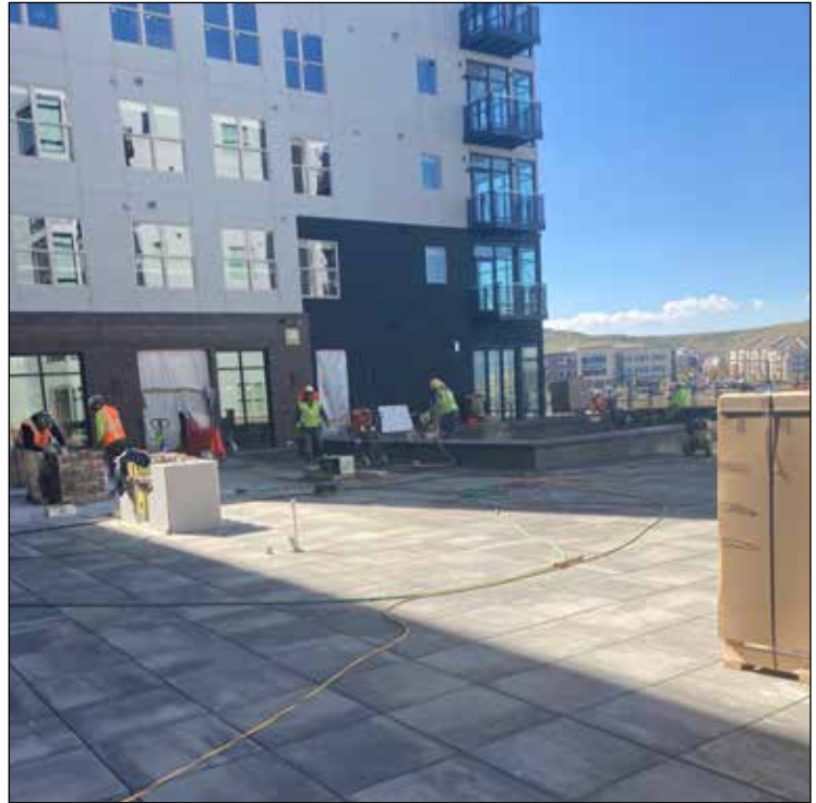
Paver installation was performed by Alpha Roofing of Denver, Colorado. Pavers covered the entire 14,000 sf rooftop area.
