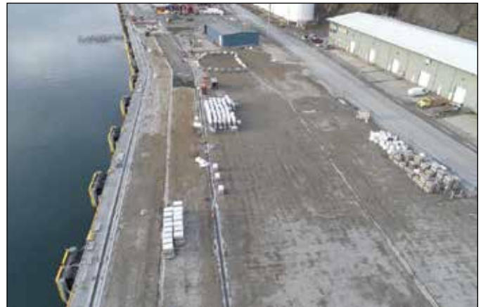
Paver installation - 90% complete | Source: PND Engineers
