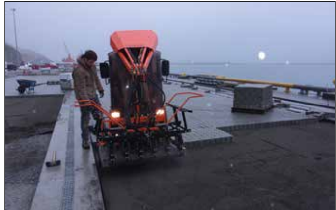
MaxLock paver pavement was installed in a herringbone pattern | Source: PND Engineers
