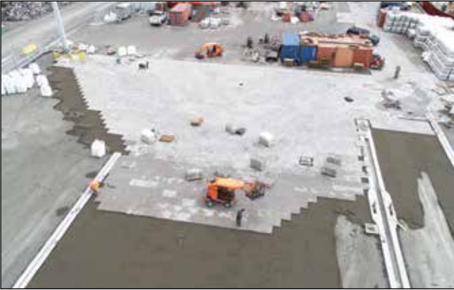
The high cost of ready-mix concrete for the dock surface caused PND to opt for interlocking pavers | Source: PND Engineers
