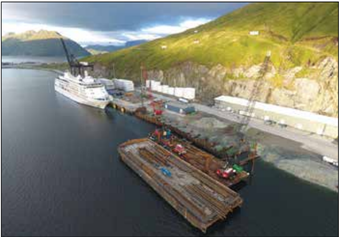
UMC, after demolition of existing facility and halfway through the construction of the Open Cell bulkhead | Source: Turnagain Marine Construction
