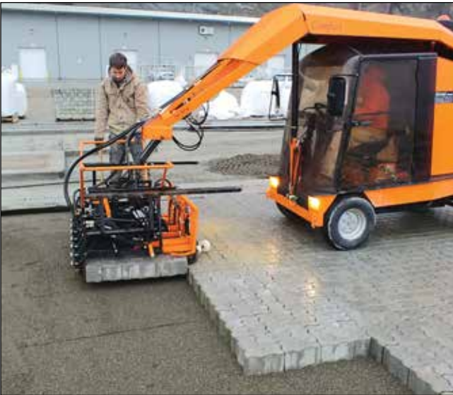
Keystone’s MaxLock pavers were the lower-cost, more efficiently installed pavement, and new to Alaska marine industries | Source: Keystone Hardscapes
